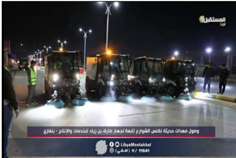
Figure 12.1 Road Maintenance in Benghazi
